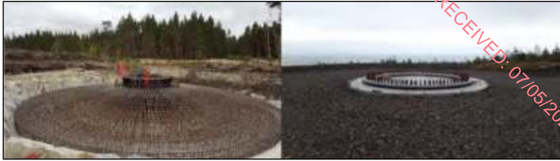
Plate 4-2 Turbine 'Anchor Cage' and finished turbine base
