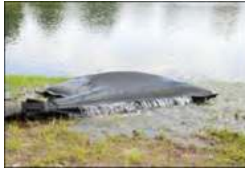
Plate 4-6 Silt bag under inspection
