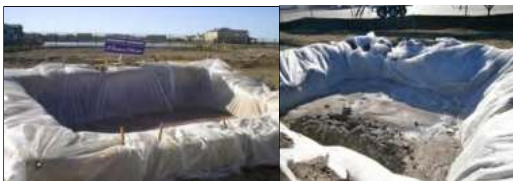
Plate 4-3 Concrete washout area
