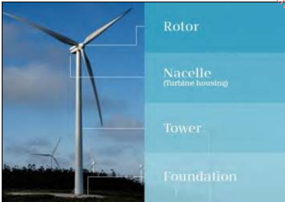
Plate 4-1 Wind turbine components
